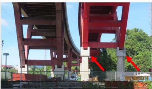
Bearing RC shear key
