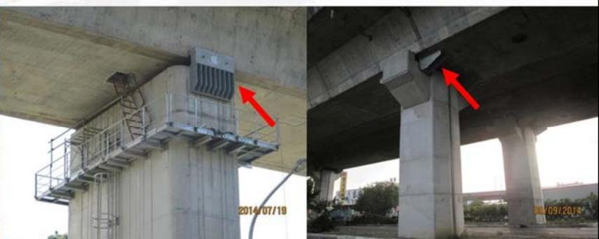
Longitudinal & transverse steel aseismic device
