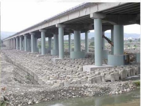
Steel jacketing on scoured piles and riverbed protection
