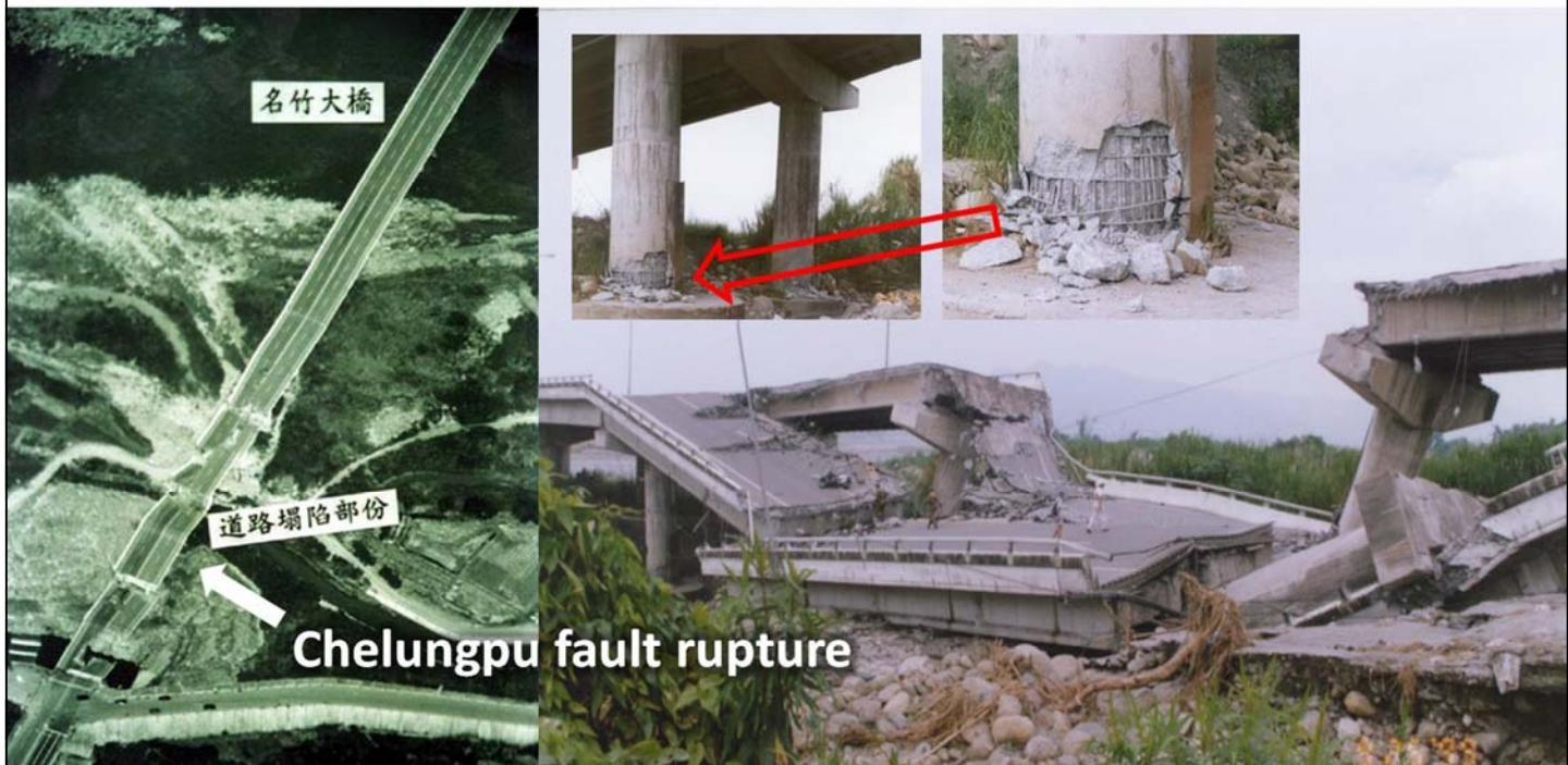
Settlement, Unseating and Shear failure of Ming-Tsu bridge,
