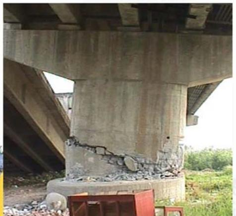
Shear failure in pier of Wu-Shi bridge, Chi-Chi Earthquake,
