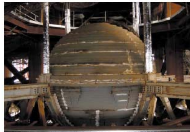
Tuned Mass Damper (被動調諧質量阻尼器) (Taipei 101)
