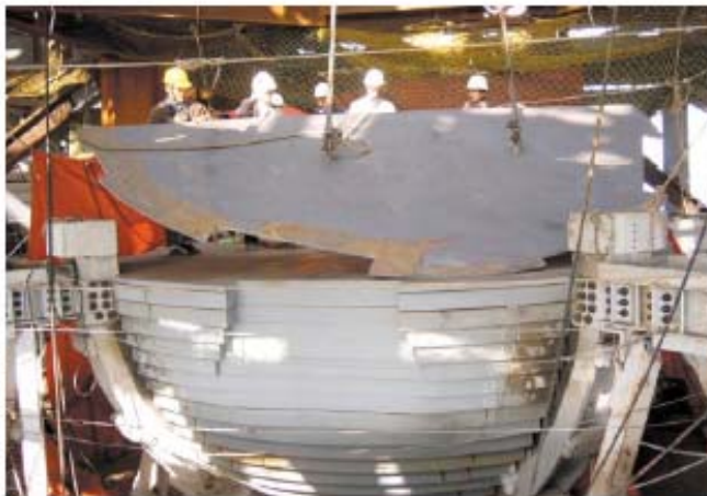
Tuned Mass Damper (被動調諧質量阻尼器) (Taipei 101)
