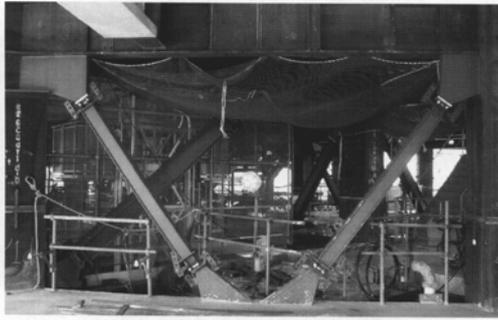
Fig. 6 Photo of buckling-restrained brace installed on site
