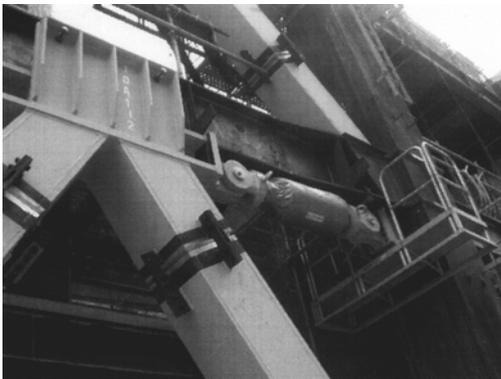
Fig. 21(b) Installed oil damper
